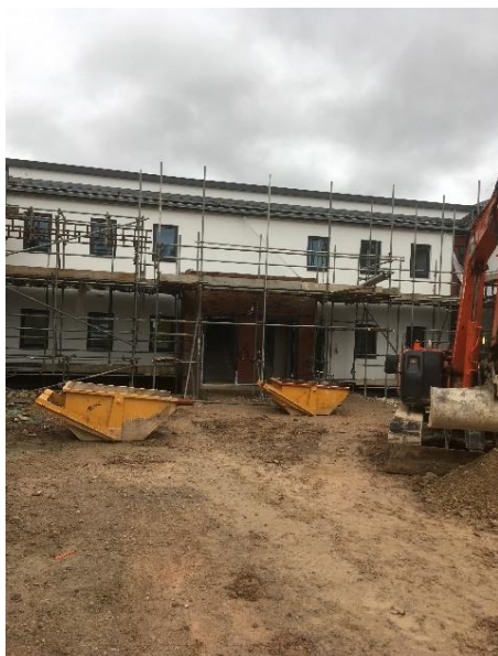
Figure 4: Awel Y Dyffryn, Denbigh Extra Care units under construction
